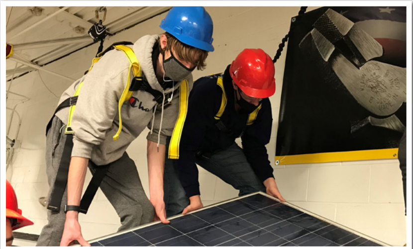
From left, Residential and Commercial Electrical students Brandon Barker (Brockport) and Eric Woodams (Kendall) install solar panels during a collaboration with the BOCES 2 Operations and Maintenance Department.
